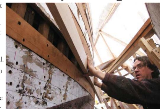
Shipwright and former *Thelma C* owner Brian Johnson fitting a new plank into the port side hull of the *Thelma C*, April, 2012
