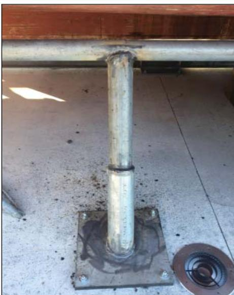
*Thelma C cradle, showing a pylon attached to the rail supporting the hull. Photo: KMM*
