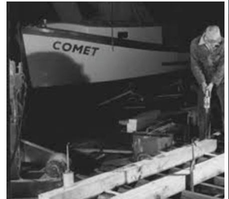
Chuck Wells, future owner of the famed crabber Shaman, drilling engine mount holes for his new gillnetter Rea in 1955.
