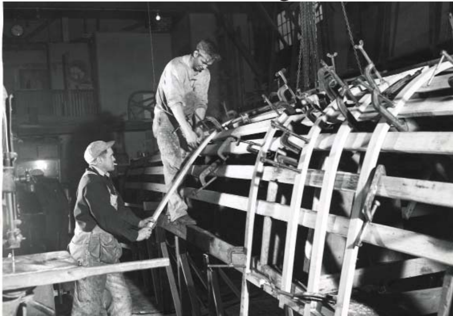
Shipwrights bending ribs at Commercial Marine Construction, 1955. Photo: Suzanne Dills
